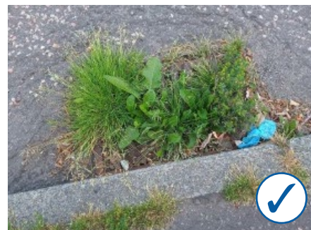
Gully blocked with vegetation
